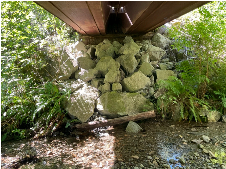
Right Bank Abutment when facing downstream
