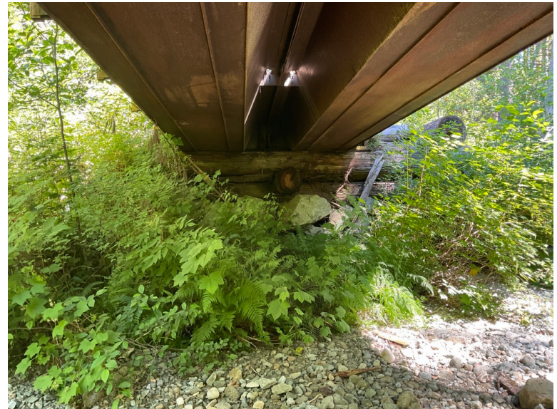
Left Bank Abutment when facing downstream
