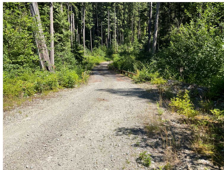
Approach from Right Bank when facing downstream
